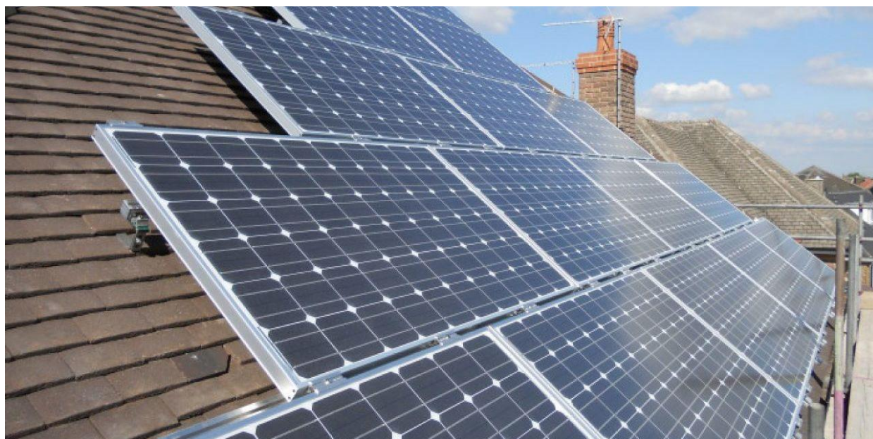
Figure 17: Micro PV installation
